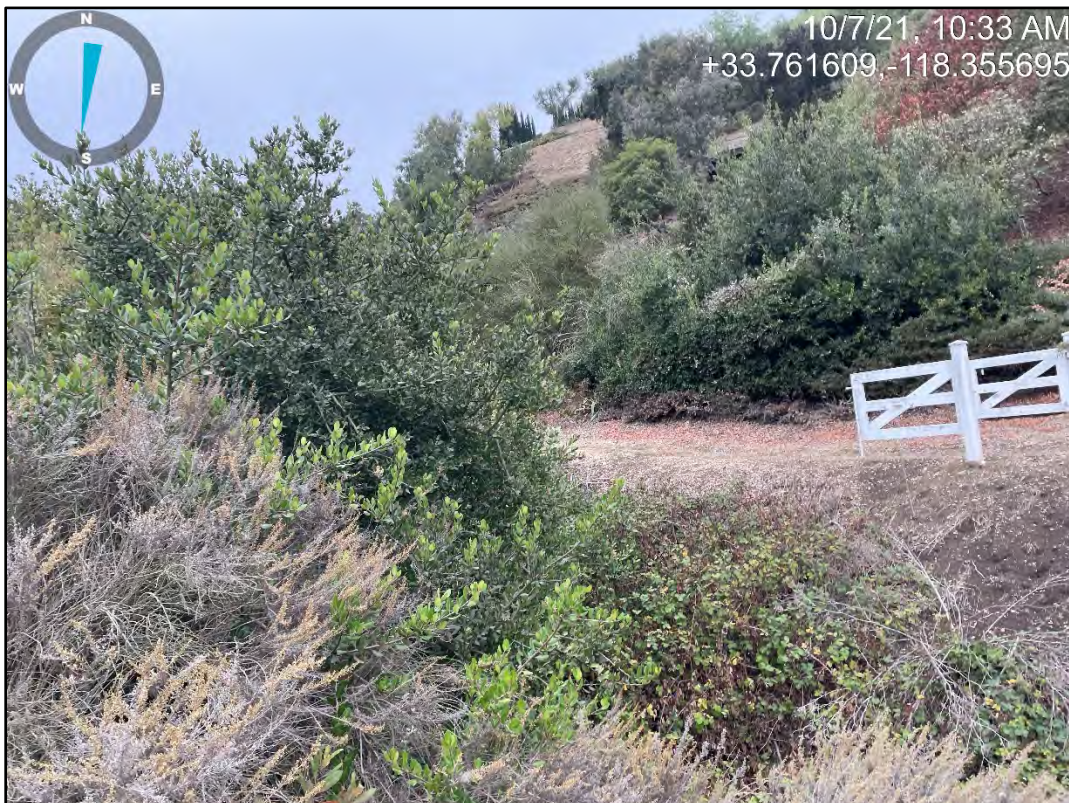
Photo 4. Rear View of 4 Quail Ridge Road North
