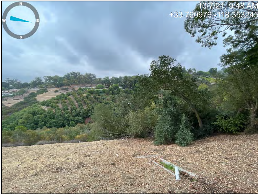
Photo 1. Rear View of 7 Quail Ridge Road North
