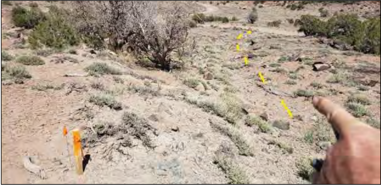
Figure 35: Another photo of GDH2, showing the reclaimed access alignment represented by yellow dashes. Wood and rocks that were scattered across are still visible, though vegetation is mature and would be considered complete.
