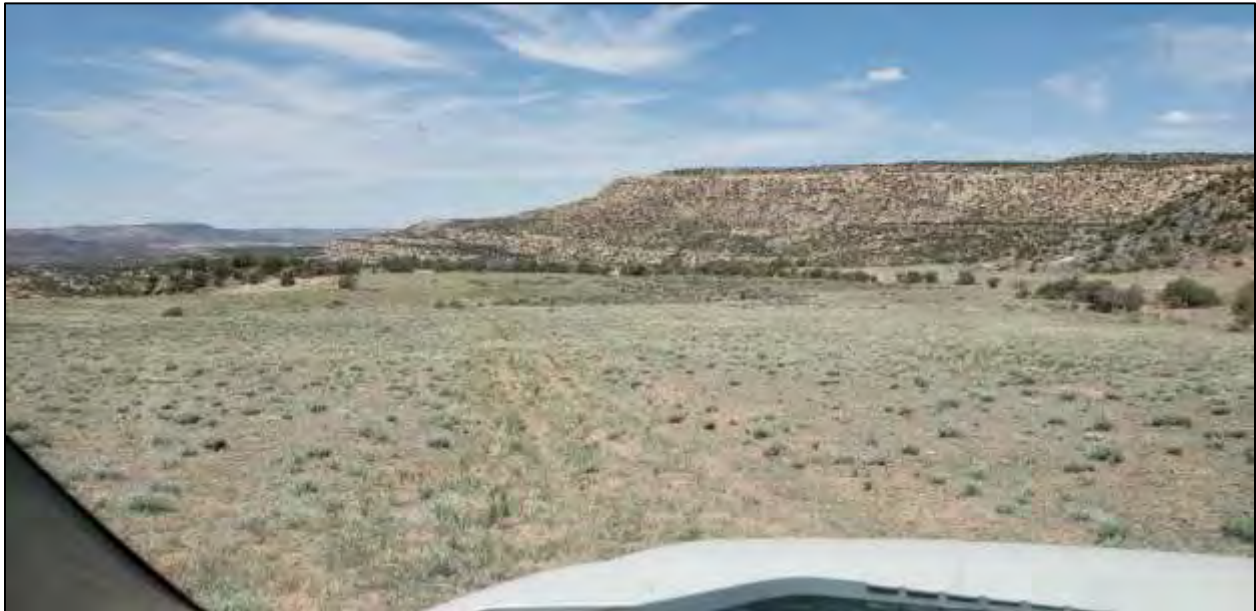
Figure 7: The roadway, taken just past the previous photograph, near sites SDH10 and SDH11. Note that the wheel tracks are very faint in this location. Care should be taken to minimize the number of times this site is driven across, to keep the ruts from getting more incised. The ruts should be raked and seeded, and brush scattered across where practical. Some sort of barrier (boulders, logs) should be placed across the road south of this location at a topographic choke point to prevent UTV's and ATVs from driving up and down and making this a permanent roadway.
