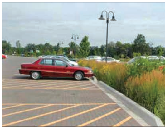
Interlocking concrete pavers with curb inlets to direct rainwater to bioretention area
