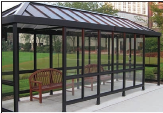
Bus Shelter to promote Public Transportation
