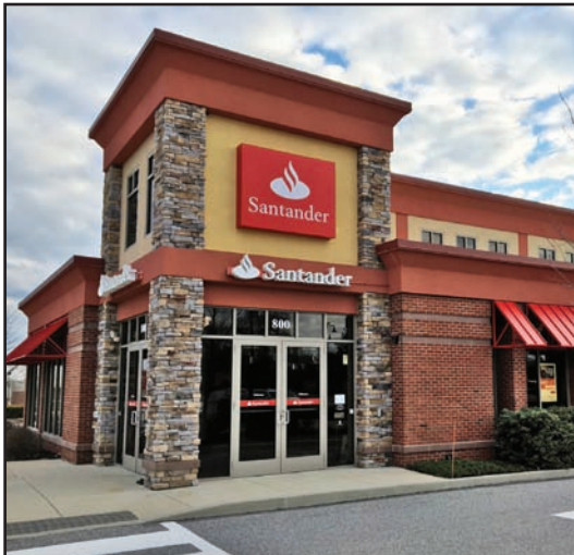
Two-Story Building with varying and complementary materials and colors
