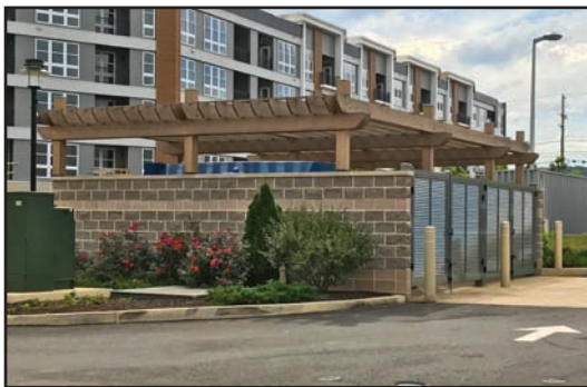
Dumpster screened inside enclosure
