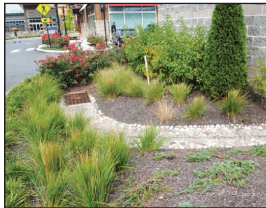
Stormwater infiltration system in parking area
