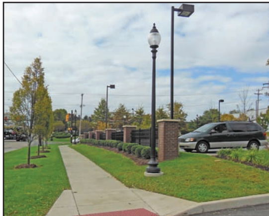
Parking screened with Pier-Fence-Hedge- Street Tree combination
