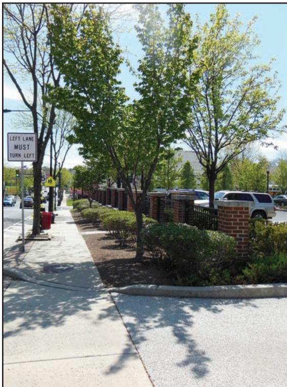
Pier-Fence-Hedge screening parking lot
