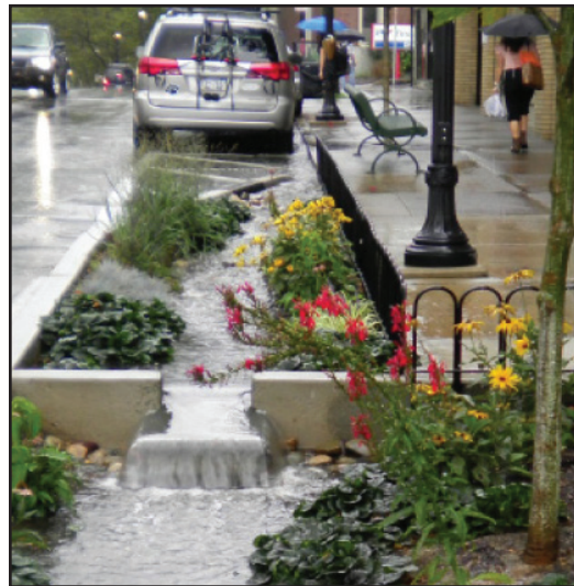
Bioswale along street providing Stormwater Management
