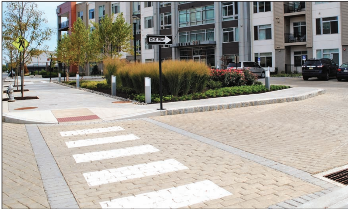
Concrete pavers and Belgian Block curbing used to enhance parking court
