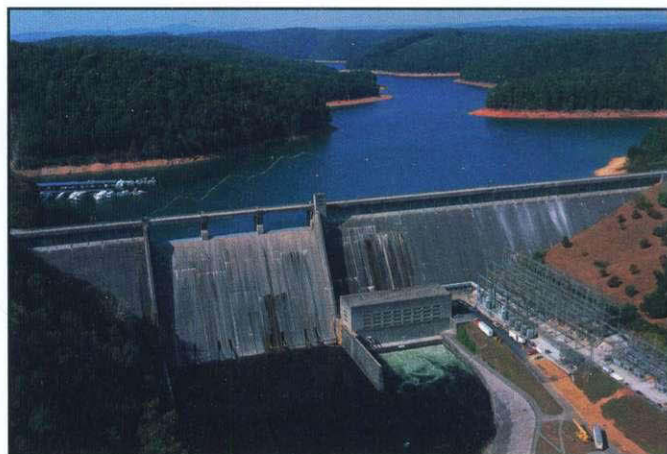
Norris Dam on the Clinch River, Tennessee, the first large dam built by the Tennessee Valley Authority in 1936. Large dams fragment populations, impede migration of fishes, and are points of introduction for many nonindigenous fishes.
