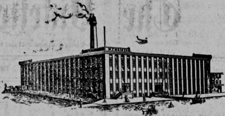
THE W. F. MAIN CO. FACTORY UNDER PROCESS OF COMPLETION AT IOWA CITY, IOWA. This completed will be the Largest Jewelry Factory in the United States (containing over 55,000 feet of floor space) and the only one located in the West.
