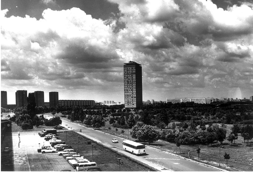
Figure 9.7 Block 16 with the League of Communists of Yugoslavia headquarters, late 1960s. Source: Belgrade City Museum.
