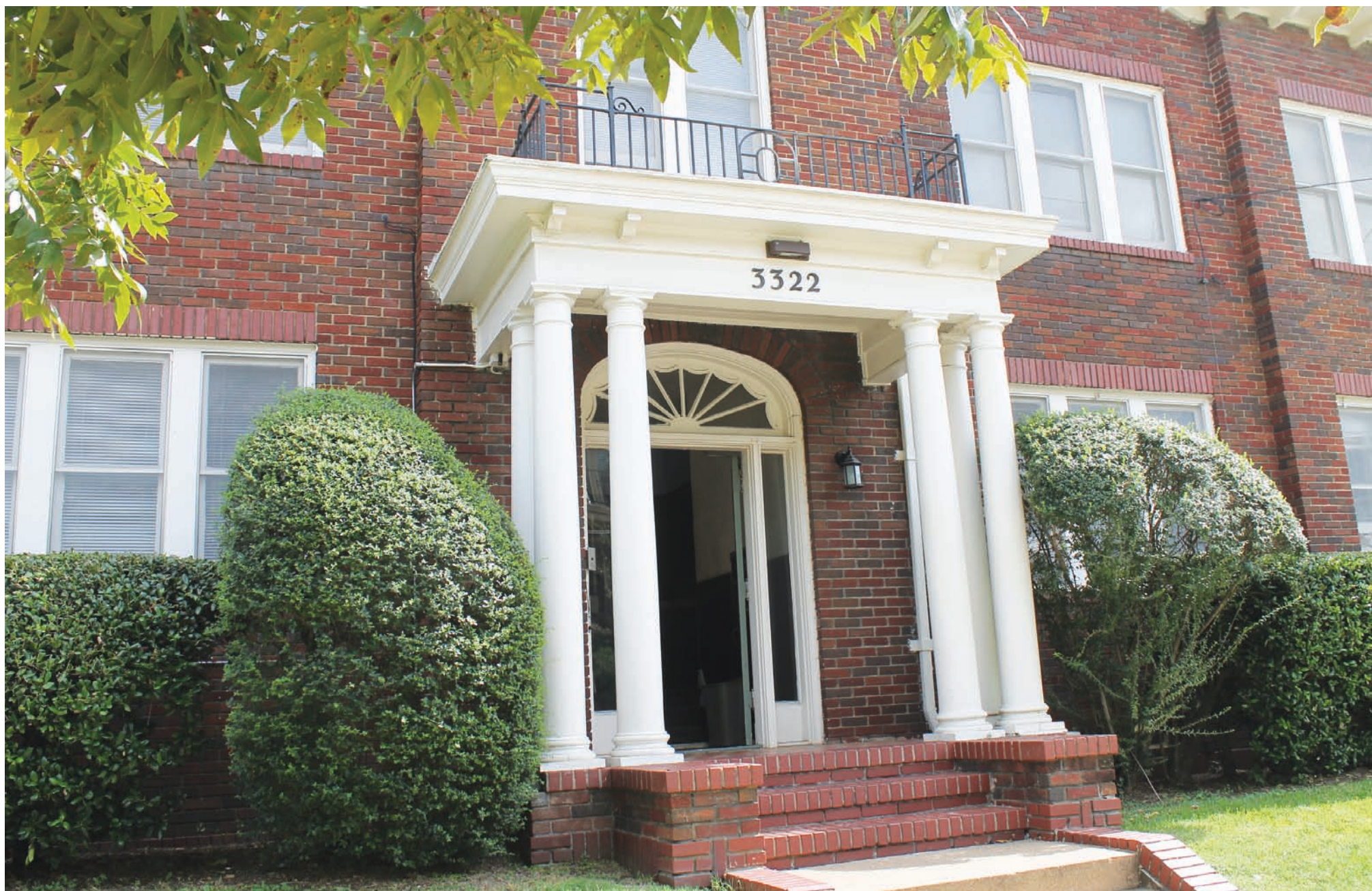
BRICK-A-BRAC | Historic buildings in Oak Lawn, like this 90-year-old one at 3322 Knight St., has been sold and will likely be torn down to make room for more higher density developments. (David Taffet/Dallas Voice)
