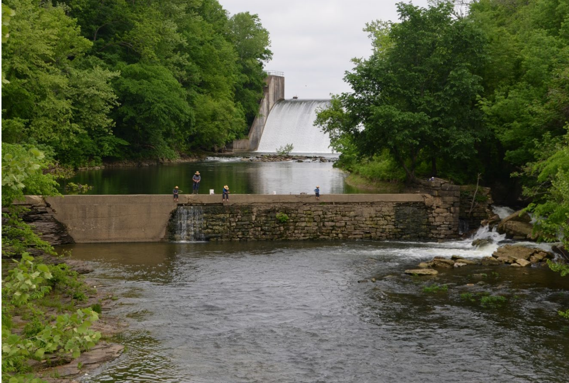
Figure 30. View of Rocky Fork Dam, a run-of-river dam forming Rocky Fork Lake, in the background, and the McCoppin Dam, a mill dam for the McCoppin Mill on Rocky Fork Creek at RM 9.1.
