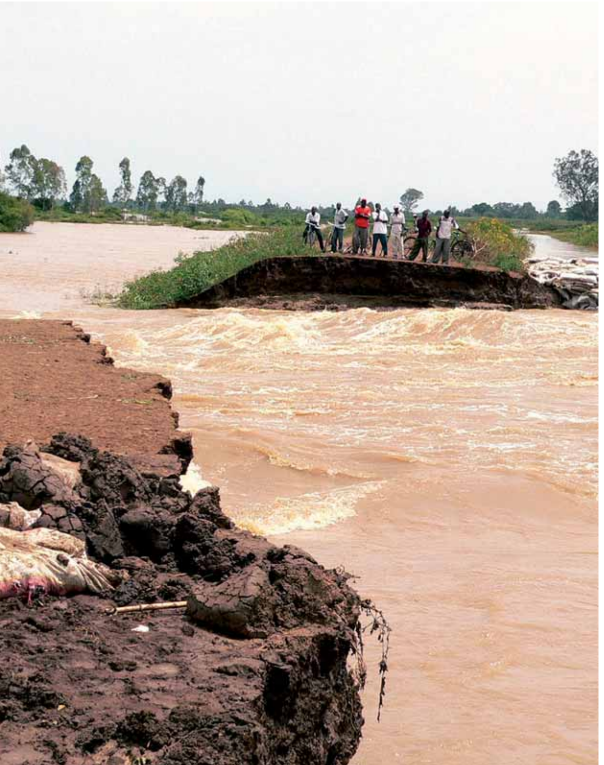
Flood waters rage through a broken dyke at Makunda in Busian, Western Kenya. Source: Edward Kale/IRIN.
