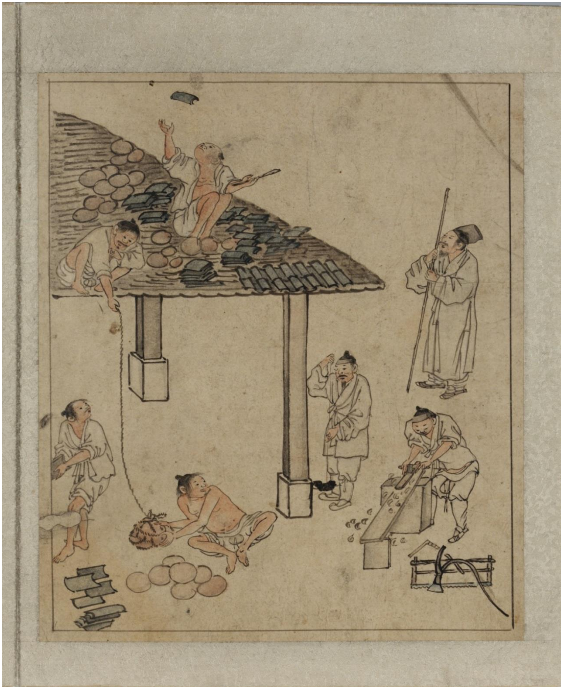
Figure 14: A crew laying roof tiles, late eighteenth century. In the bottom right, a carpenter smooths lumber with a plane while another craftsman inspects the columns. Painting by Kim Hongdo (1745-?)
