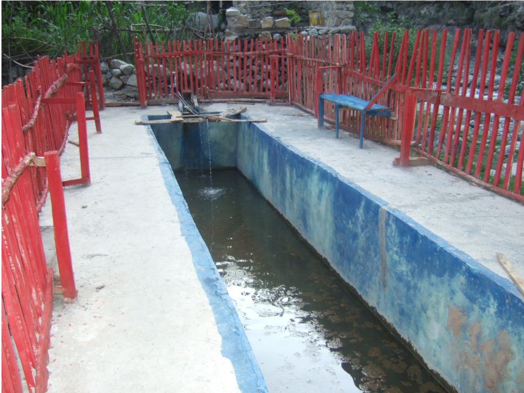
Raceway Structure on Seglo Nullah
