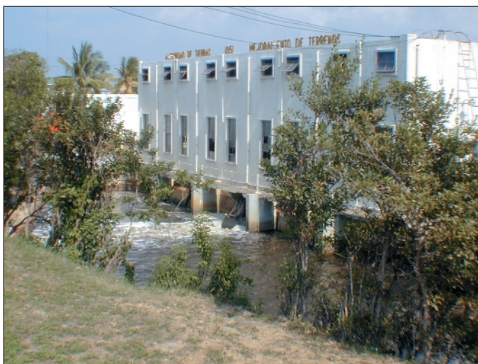
Photo 19. Pump house at Caño Tiburones, Arecibo, Puerto Rico. Photo by J. Colón.
