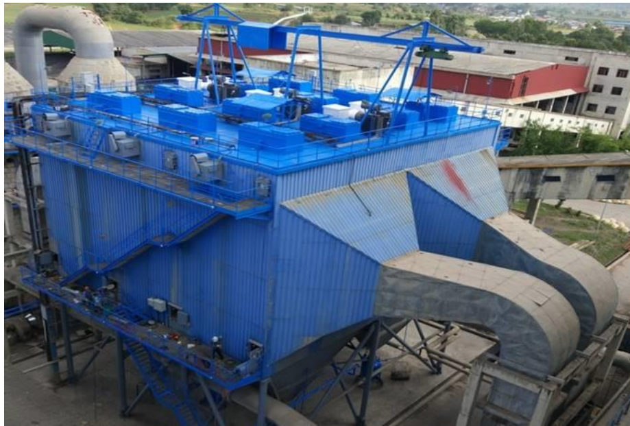
Figure 4.13 Electrostatic Precipitator (ESP)
