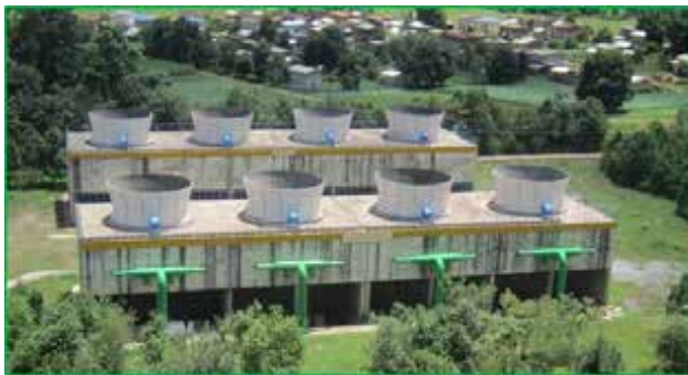
Figure 4.7 Cooling Tower of Thigyit Coal-fired Power Plant
