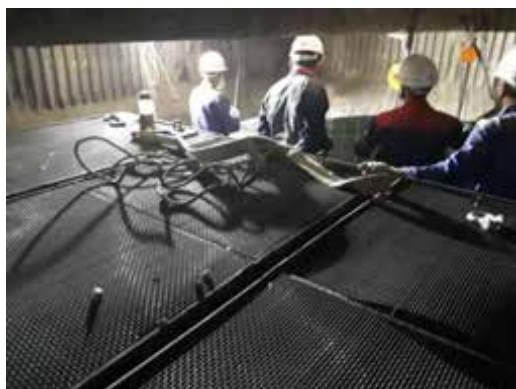
Figure 4.12 SCR system Installation
