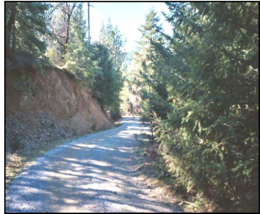
Zola Drive showing the narrow road, steep terrain, and vegetation encroachment
