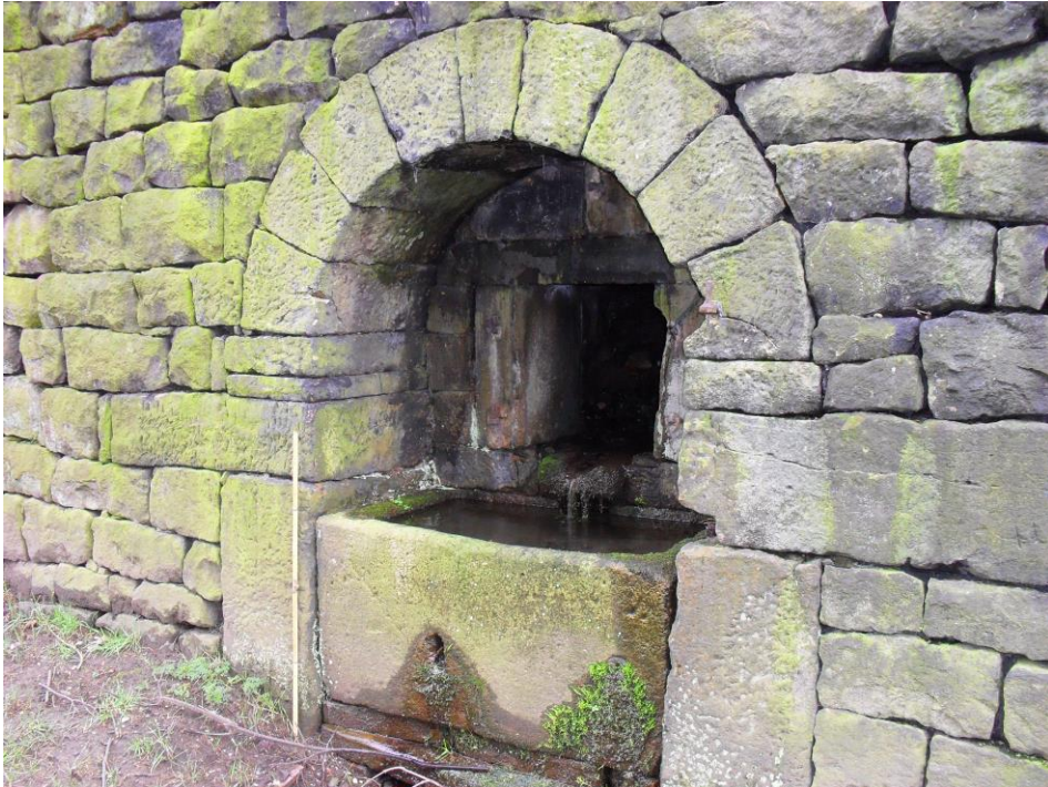
Figure 1 Large Well on Lumb Lane Almondbury. This structure is typical of many in the Pennine areas. The single block of gritstone which forms the trough is recessed into the surrounding wall and is capped by a large stone slab.
