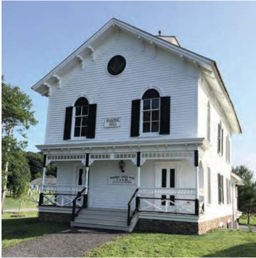
Figure 1. The Warren Masonic Lodge Number 32, Town of Clinton, Dutchess County. Photograph by Cynthia Koch.
