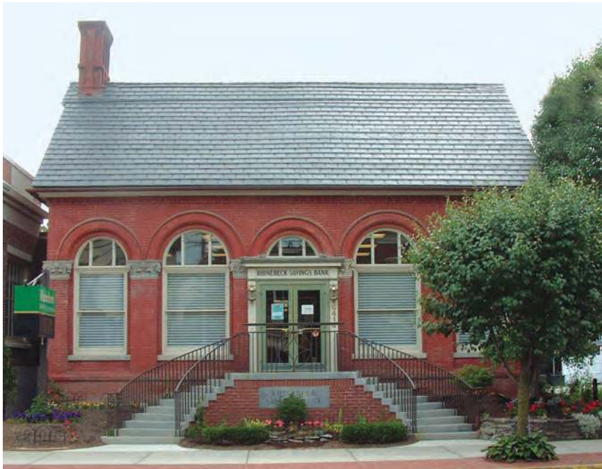
Figure 1. The original Rhinebeck Bank building , 14 Montgomery Street, Rhinebeck.
