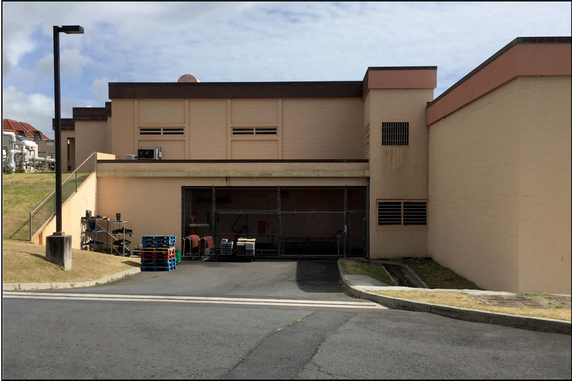
Plate 13: Phase I Addition Building (No. 04), View to North
