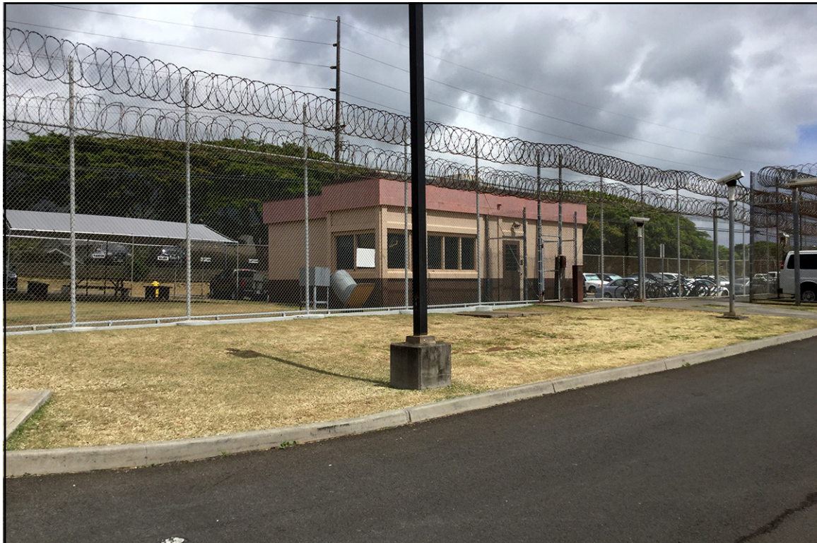
Plate 19: Gatehouse Building (No. 11), View to Northwest
