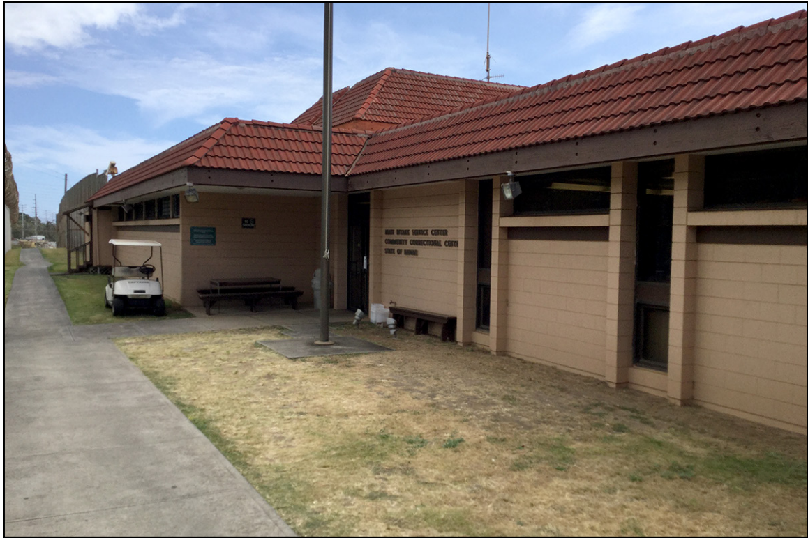
Plate 15: Intake Service Center Building (No. 05), View to North
