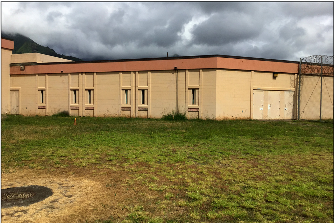
Plate 12: Module C Housing Building (No. 03), View to Northwest
