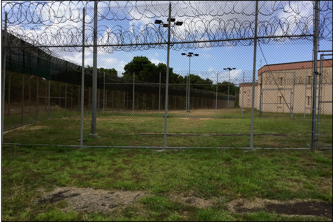
Plate 2: Open Yards East of Modules A, B, and C, View to South
