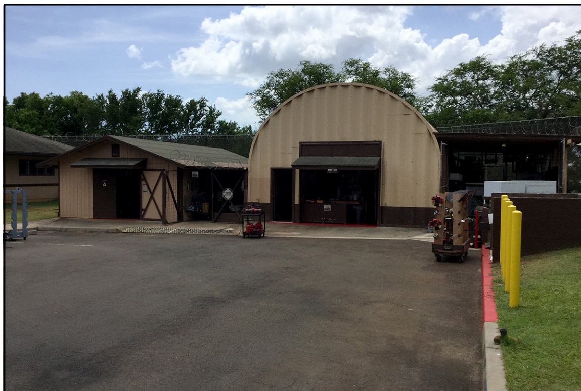
Plate 18: Maintenance Shop Buildings (No. 12B, left, and 12C, right), View to Northeast
