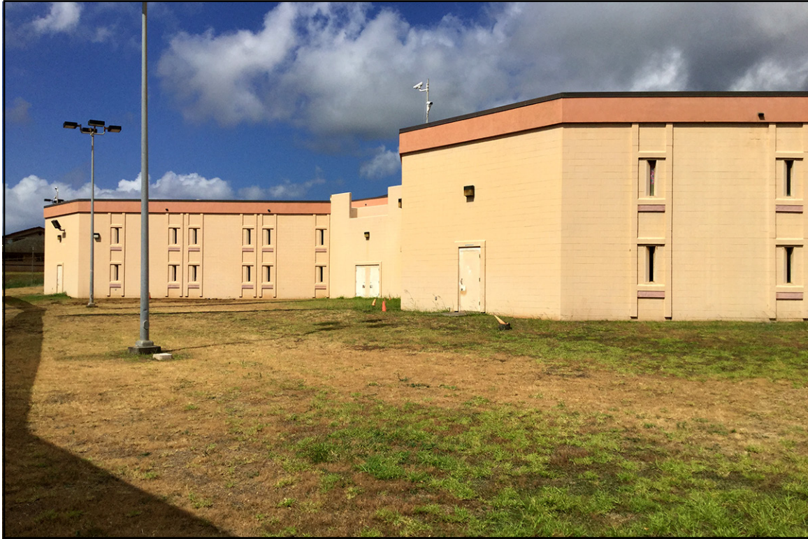
Plate 11: Modules A and B Housing Buildings (No. 01, right, and No. 02, left), View to Southwest
