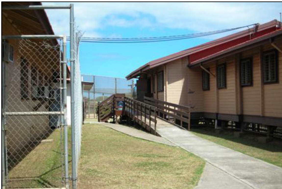
Plate 5: Housing Building (No. 07), View to North
