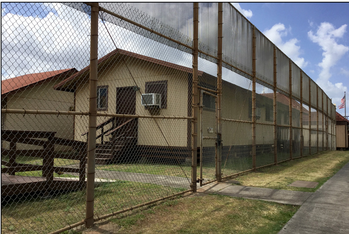
Plate 7: Training Building (No. 13), View to Southeast
