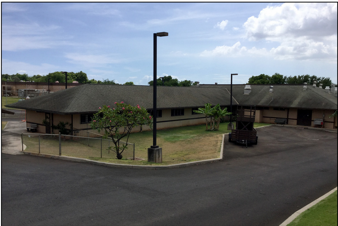
Plate 16: Low Custody Housing Building (No. 12A), View to Northeast
