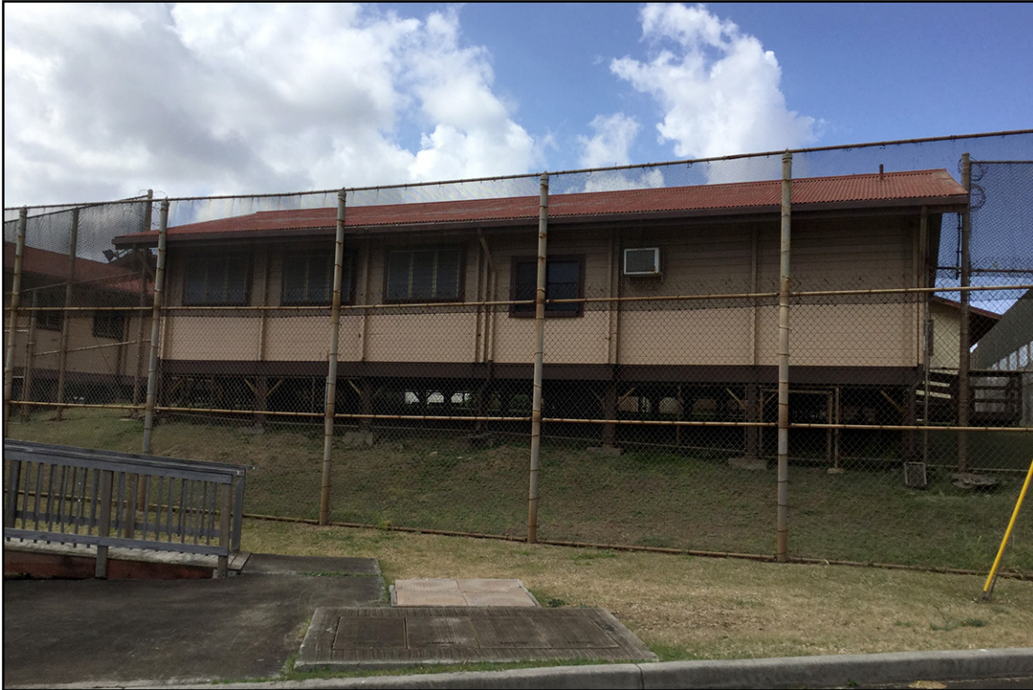
Plate 4: Program Building (No. 08), View to South
