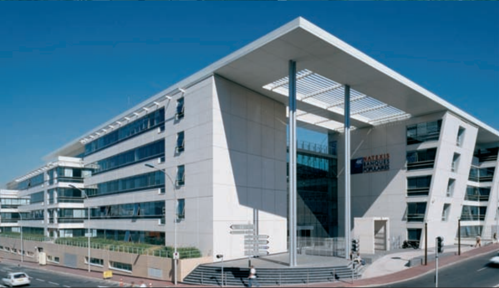
Top. Standing alongside the Bercy park in Paris (12 th arrondissement), the Bercy Parc complex comprises 110 housing units, three shops and a day-care centre.
