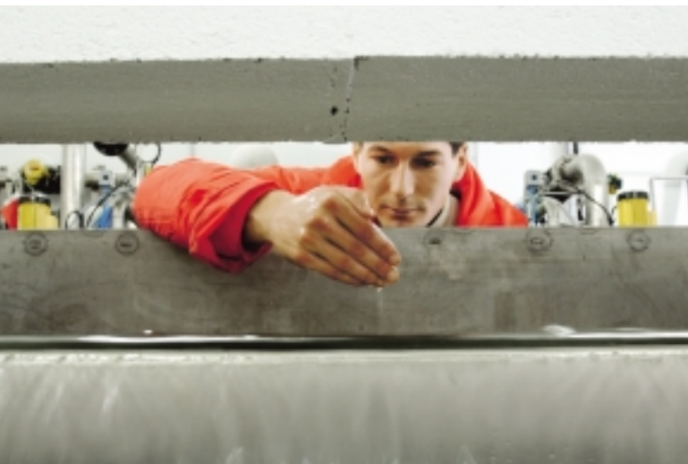
Water treatment station, Rambouillet factory, France.
