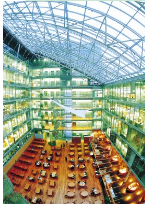
The new Nokia House in Espoo Finland is covered with a unique eco-facade, an extra layer of glass to idealize the temperature inside.
