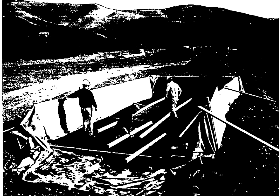
CONSTRUCTING UNDER-DRAINS looking north, 6/15/96 Fig 20
