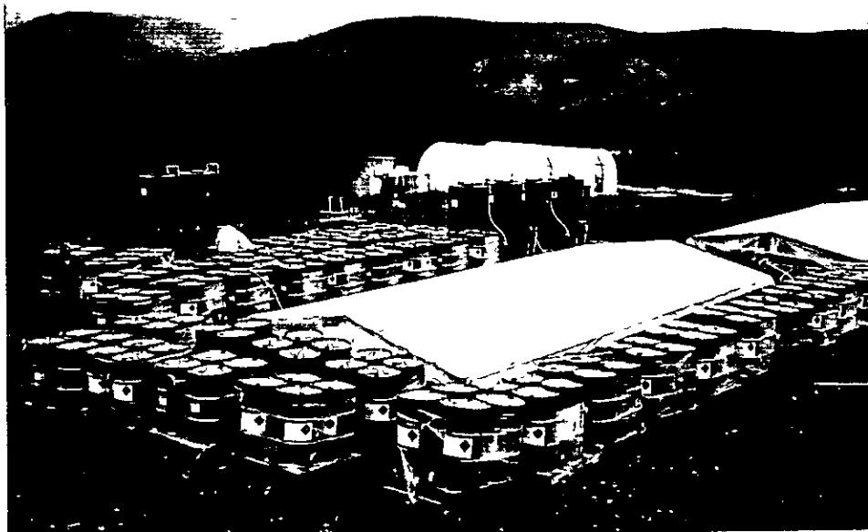
INITIAL LOADING OF SOLVENT INTO CLEAN SOLVENT CELL looking south, 6/20/96 Fig 26
