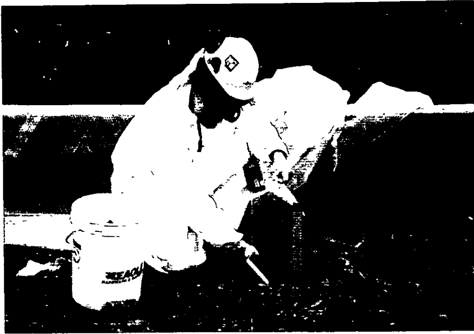
CONFIRMATION SAMPLING AT SURFACE OF CELL looking west, 8/1/96 Fig 28
