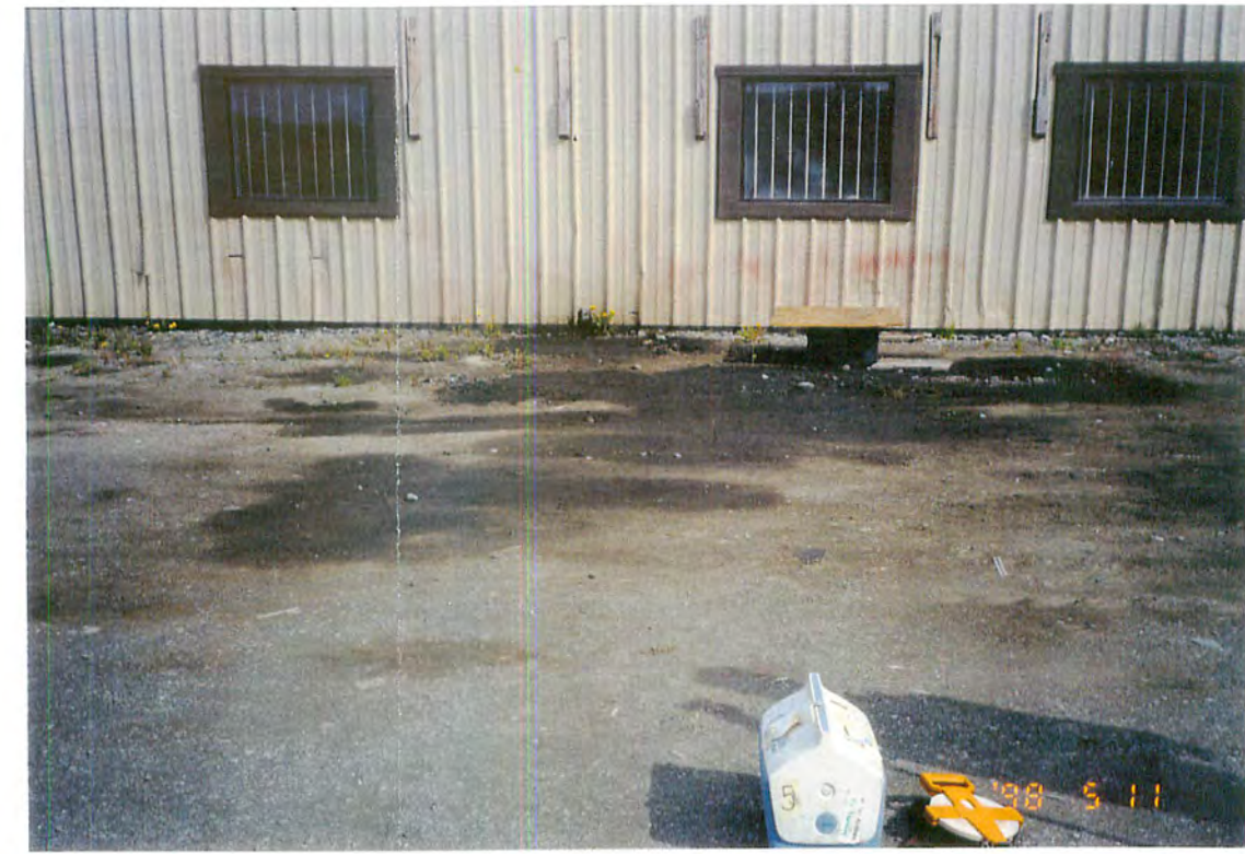
FIGURES 7 & 8: VIEWS OF A USED OIL SPILL NEAR THE SOUTHERN END OF THE FACILITY. THE MOST HEAVILY STAINED PORTIONS COMPRISE AN AREA EXCEEDING 250 SF, WITHIN A STAINED AREA APPROXIMATING 1900 SF.
