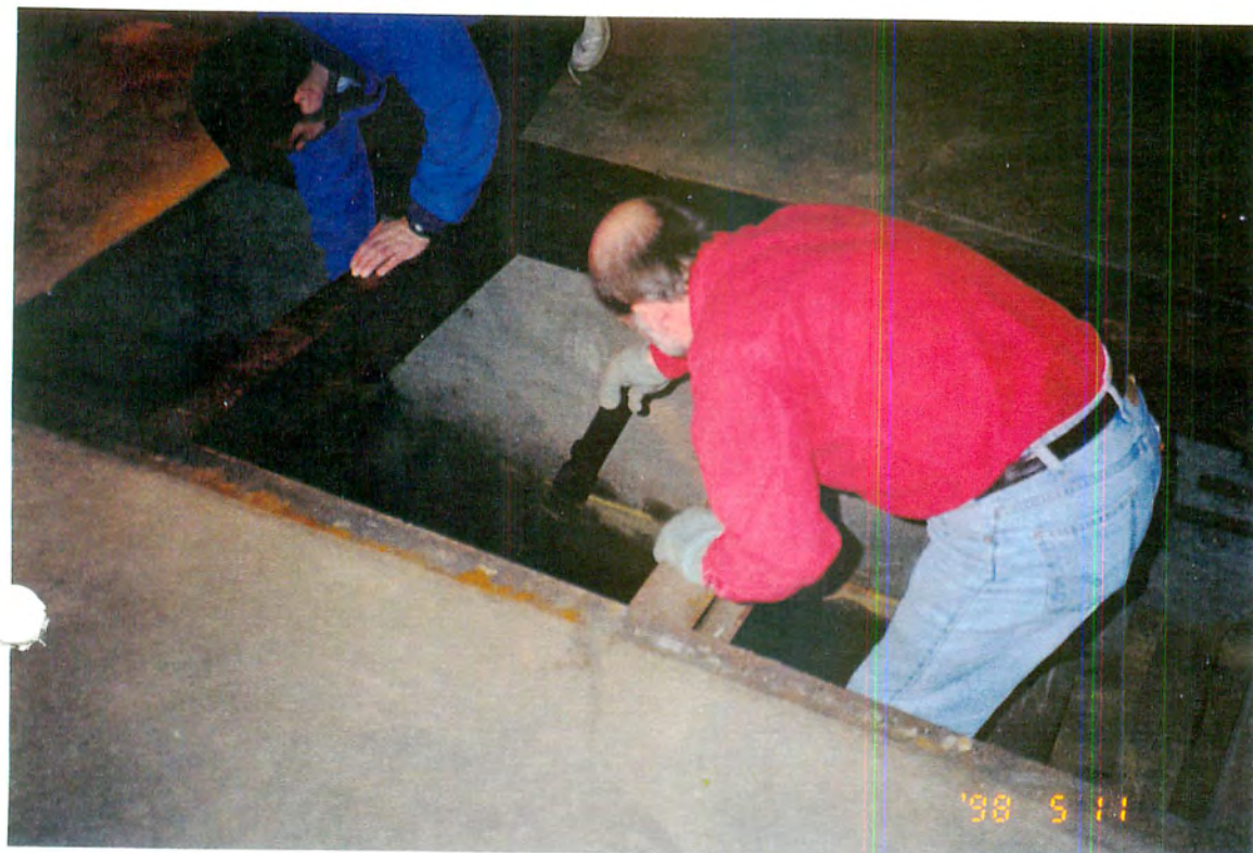
FIGURES 9 & 10: NORTH GREASE PIT (DESIGNATED "B-1" BY JMM). NOTE SUMP IN FLOOR OF PIT (PHOTO 9). 5 IN CAST IRON PIPE EXITS THIS PIT FROM WEST WALL, TERMINUS UNKNOWN.
