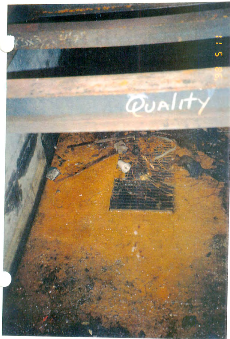
FIGURES 9 & 10: NORTH GREASE PIT (DESIGNATED "B-1" BY JMM). NOTE SUMP IN FLOOR OF PIT (PHOTO 9). 5 IN CAST IRON PIPE EXITS THIS PIT FROM WEST WALL, TERMINUS UNKNOWN.
