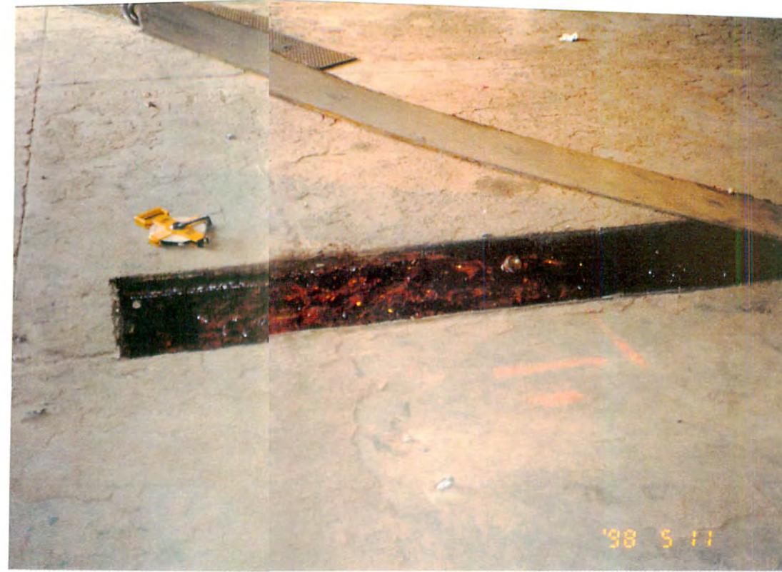
FIGURES 11 & 12: DRAINAGE SUMP B-5 IN SOUTH BAY (FORMER PAINT SHOP). PAINT WASTE EVIDENT IN SUMP CONTENTS; JMM VERIFIED HAZARDOUS LEVELS OF HEAVY METALS IN SUMP SLUDGES.
