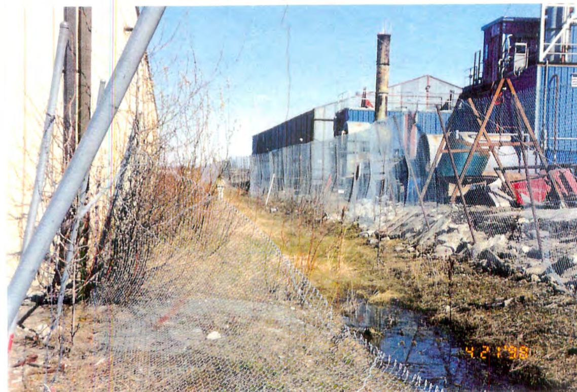
FIGURE 2: EASTERN PROPERTY LINE OF SUBJECT FACILITY AND GENERATOR AT ADJACENT EITECH COMPLEX.
