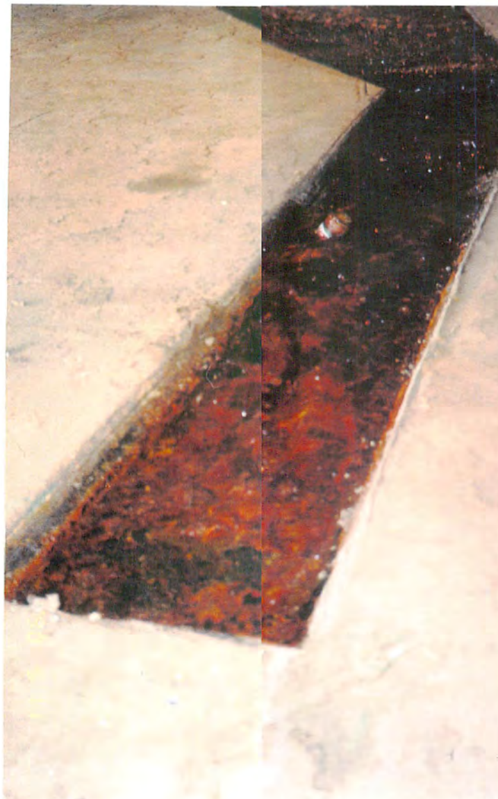
FIGURES 9 & 10: NORTH GREASE PIT (DESIGNATED "B-1" BY JMM). NOTE SUMP IN FLOOR OF PIT (PHOTO 9). 5 IN CAST IRON PIPE EXITS THIS PIT FROM WEST WALL, TERMINUS UNKNOWN.
