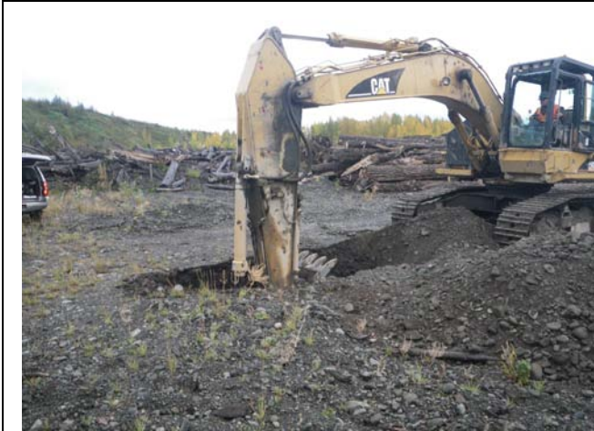
Photo 1. Excavating test pit 01 (looking north)
