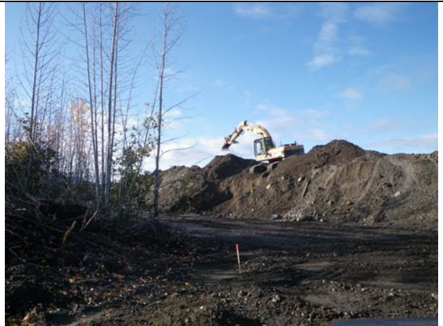
Photo 20. Moving overburden to access test pit 23 (looking north)
