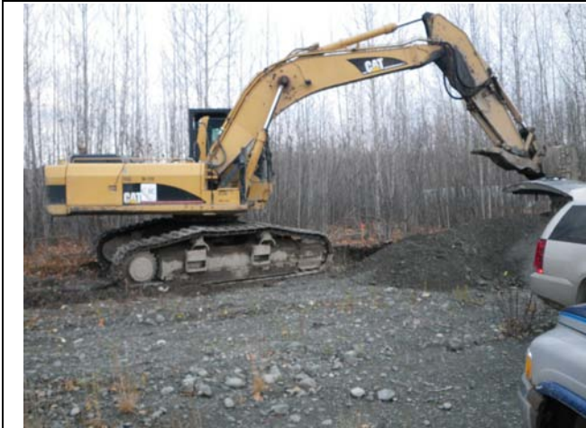
Photo 25. Excavating test pit 34 (looking east)
