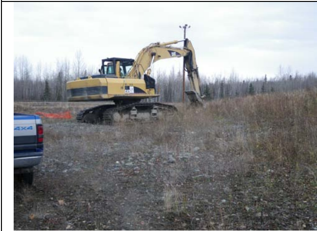
Photo 27. Test Pit 39 (looking northwest)
