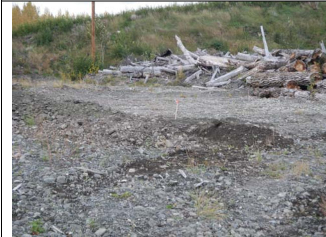
Photo 15. Backfilled test pit 05 (looking north)
