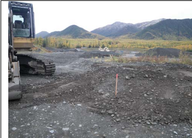
Photo 13. Backfilled test pit 02 (looking south)
