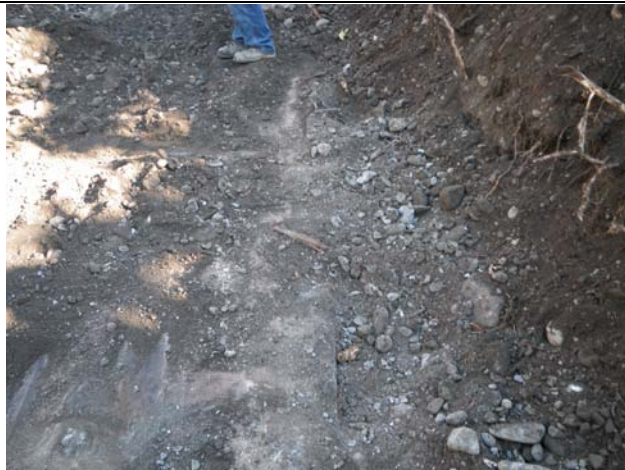
Photo 19. Concrete foundation encountered at test pit 14
