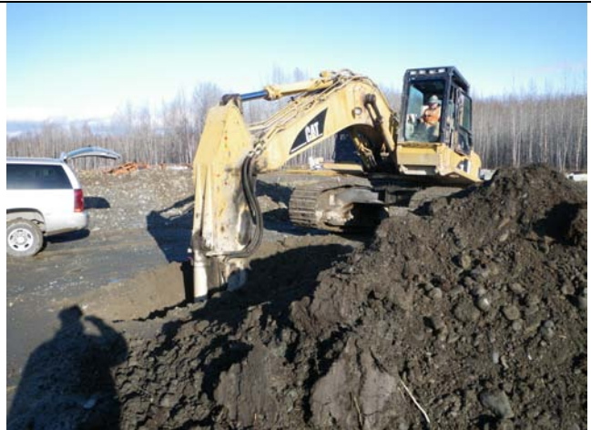
Photo 24. Excavating test pit 31 (fill material) looking north
