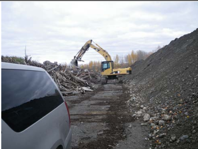
Photo 21. Moving debris to access test pit 25 (looking northeast)
