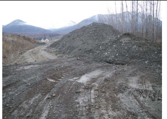
Photo 26. Backfilled test pit 38 (looking southeast)
