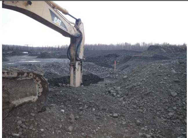
Photo 22. Excavating test pit 26 (looking west)
