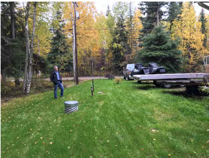
Photo 2: Underground storage tank and culvert (Facing west)
