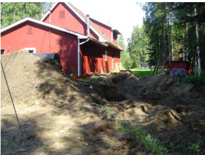
Photo 3: Site Excavation photo (Facing east, predating 2018)
