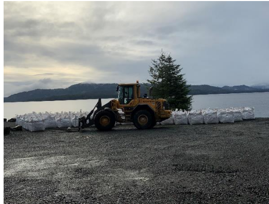
Excavation of Petroleum Contaminated Soil, Discovery Campus, Kasaan
