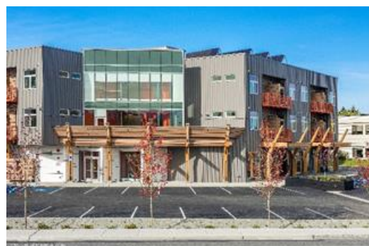
Mixed Use Development of Former Gas Station, Alpina Site, Anchorage
