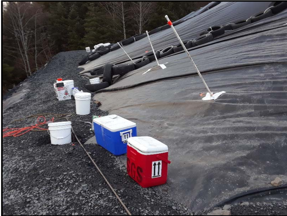
Photo 1: Looking northwest at the pore water sampling points installed in the southwestern corner of the treated stockpile at the former Byford Junkyard Site.
