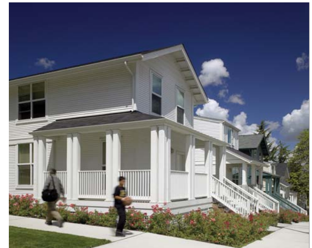
The Hope VI program replaced many distressed projects with new mixed income neighborhoods.
