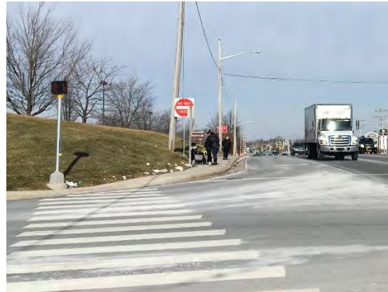
Riders waiting for bus at US 202 / SB Rocky Run Parkway stop
