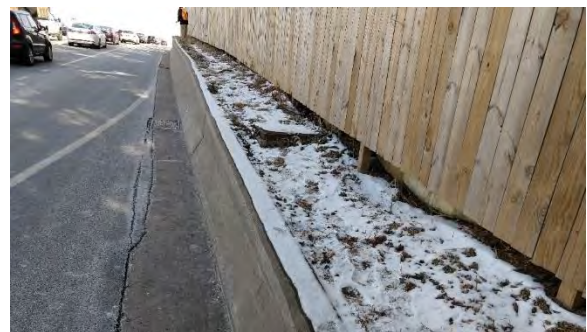
Missing sidewalk at Widener University
