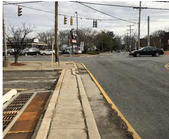
North side of Brandywine Blvd
