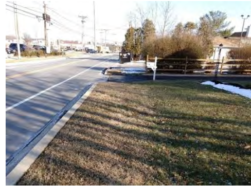
Missing sidewalk on Garden of Eden Rd
