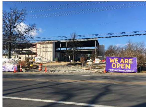
YMCA under construction
