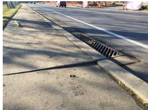
Elevation difference near inlet
