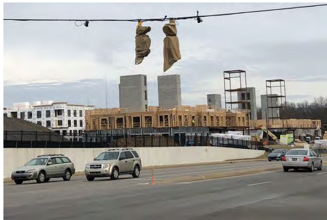
Concord Plaza under construction
