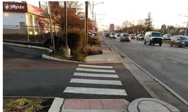
New crosswalk installation at Seasons Pizza
