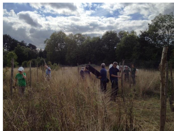
Horton Country Park LNR Countryside team volunteers erecting deer fencing in Lambert's Orchard late summer 2015
