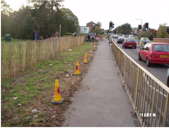
Hogsmill Local Nature Reserve Ruxley Lane 2006 with wider easier to maintain grass verge and new hedge with temporary fence
