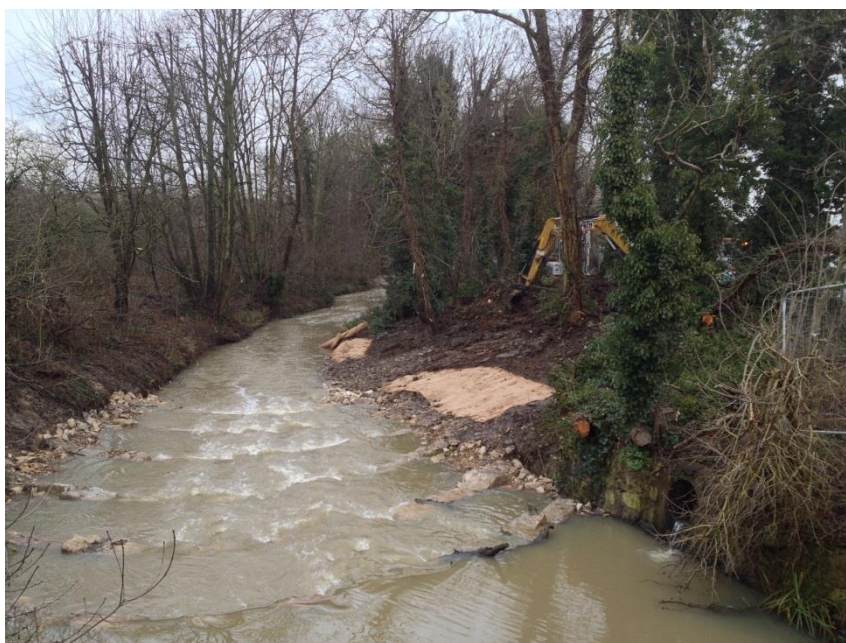
Rock ramp by the A240 Bridge late winter 2015
