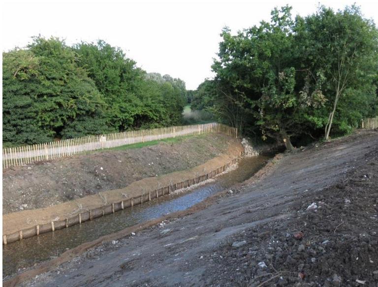
Hogsmill LNR former location of weir just after removal summer 2013
