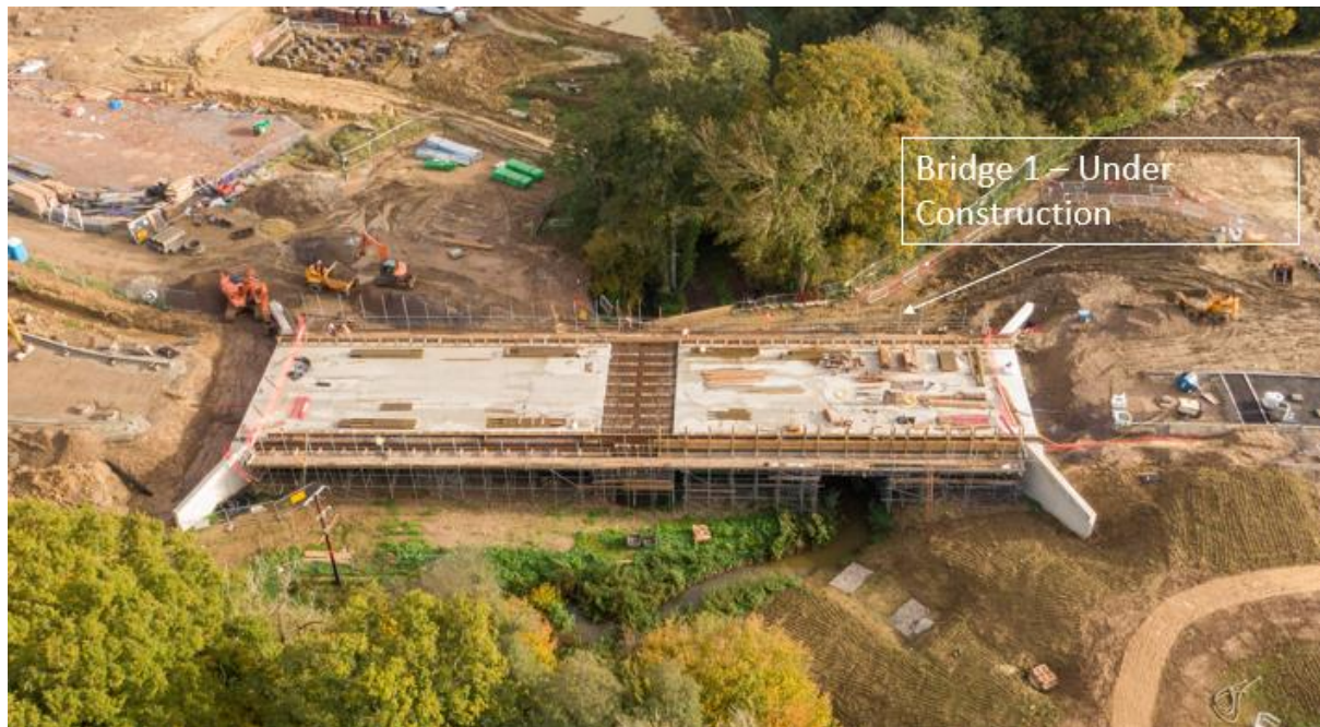
Plate 7: Bridge 1 Progress @ 31 Oct 2020
