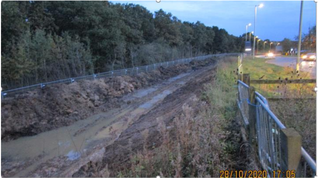
PLATE 10: View of Embankment Works from R3 looking South 28 Oct 2020
