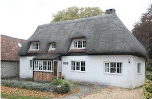
Figure 16: Conservation Area Building (2020).
