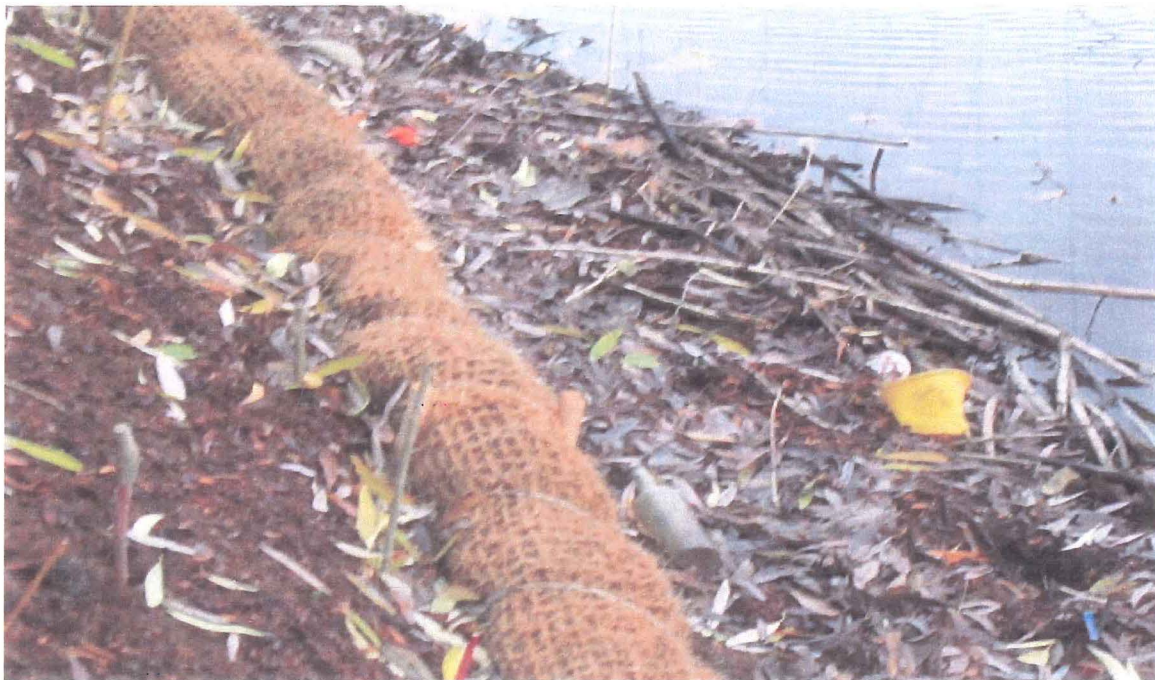
Legend 8. COIR fabric staked down on Duck Bay embankment along Lake Washington in Washington Park Arboretum.
