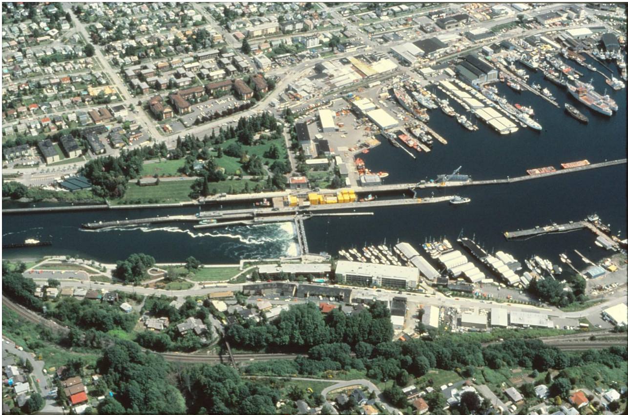
Figure 1 Aerial view of the LWSC looking north circa 1982. Locks archives
