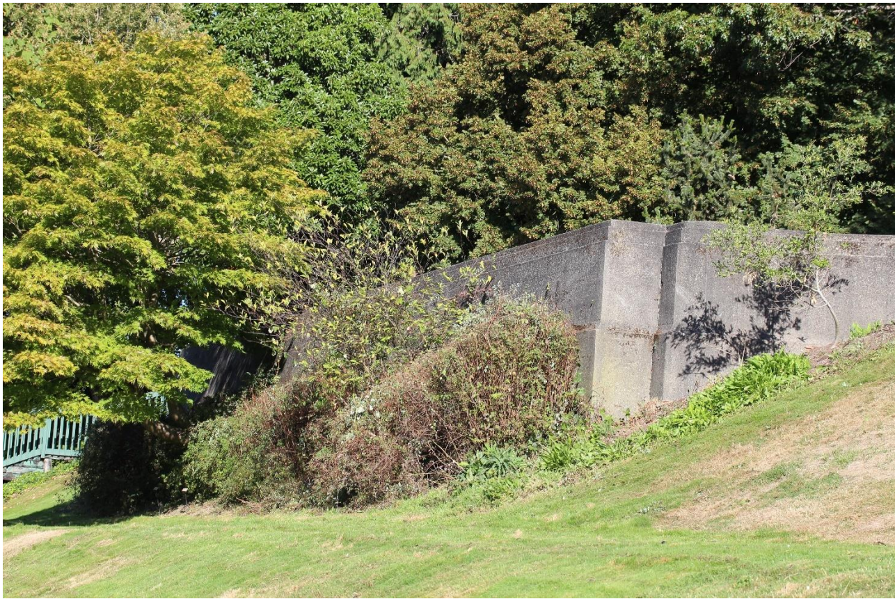
Figure 40 Bed 22 prior to renovation Summer 2016. Stephen J. Munro
