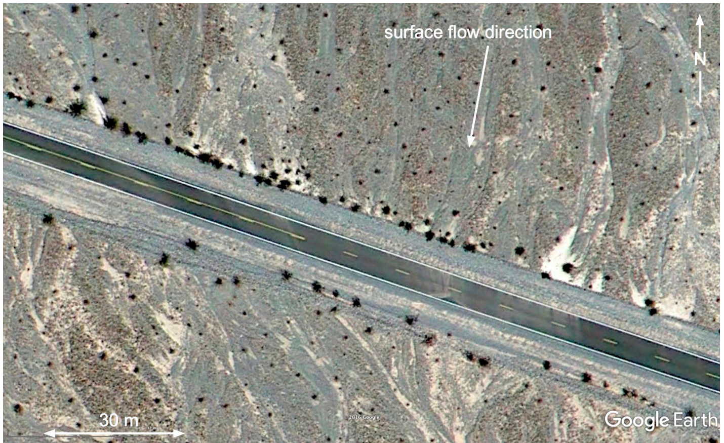
Figure 6. Google Earth image of small section of Scotty's Castle Road crossing a fan. Surface flow direction is from top to bottom. Note the enhanced creosote growth on both sides of the pavement from runoff. It is stronger on the uphill sidecast where runoff from the fan ponds into standing water as the numerous small white alkali areas show uphill of the road. Such areas are not seen downhill of downhill sidecast because there is no barrier to surface flow.
