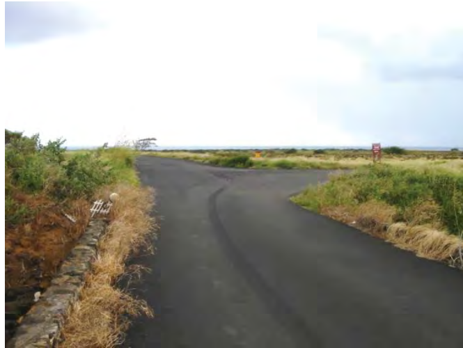
View of possible location to install the security barrier gate at South Point Road.
