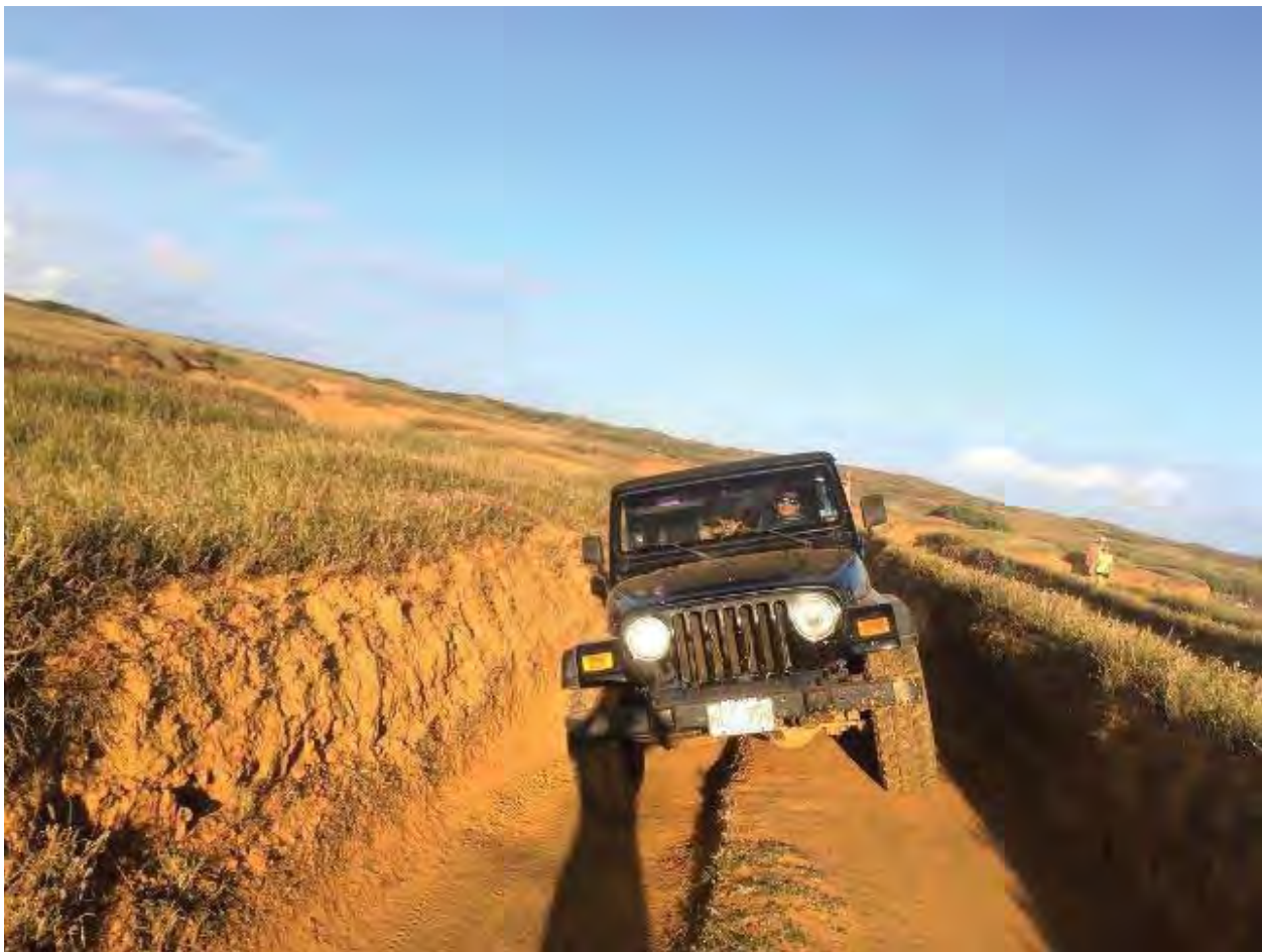
Unrestricted vehicular access at South Point has resulted in deep, wide, and extremely severe erosion scars, ranging from several feet to over eight feet in depth.
