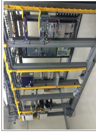
Photograph 8: Interior view of single-story structure located within the telecommunication station.
