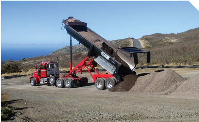
► Kahikinui Road Construction
