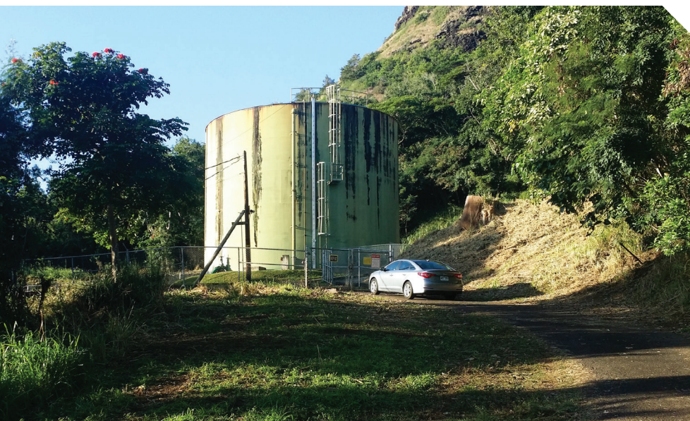
► 40-year-old Anahola Water Tank is expected to be replaced in 2021. DHHL oversees four water systems on Molokaʻi, Kauaʻi, and Hawaiʻi.
