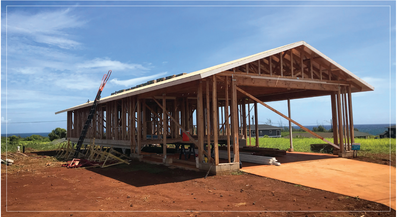
▶ Self-Help house construction in Anahola, Kaua'i
