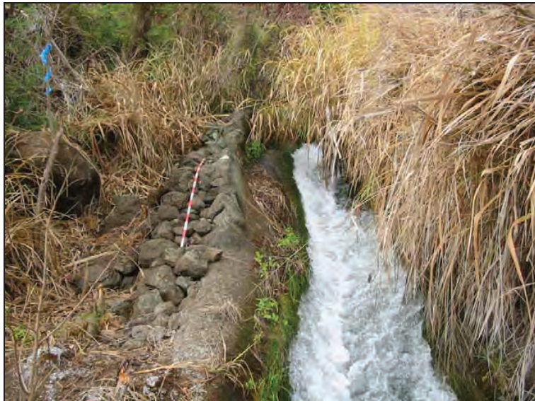
Figure 13: Site 50-50-04-5729 Ditch. View to West.
