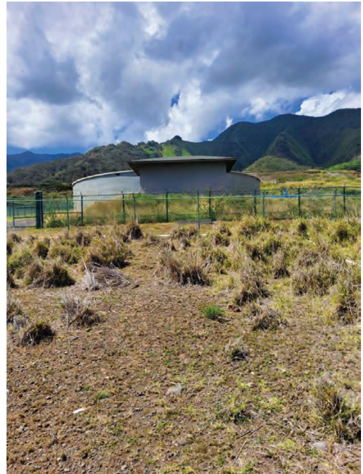
Existing County DWS 1.5-million Gallon Water Tank.
