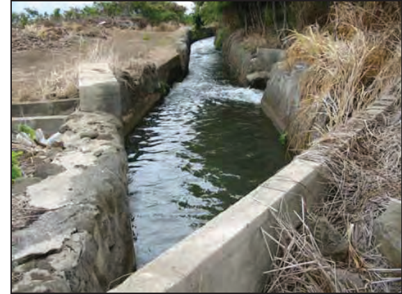
Figure 10: Waihee Ditch (50-50-04-5197). View to South.
