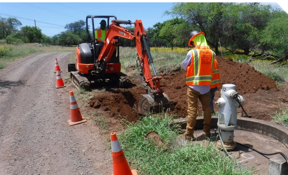
► Repair work to DHHL’s Ho‘olehua Water System on Moloka‘i
