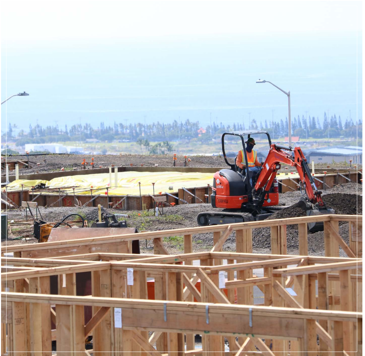
► Turnkey House Construction in Laʻfi ʻŌpua
