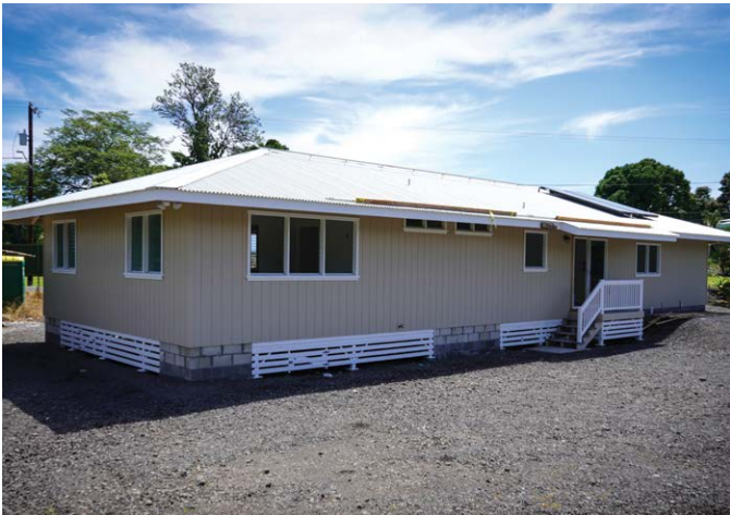
▶ Hawai‘i Community College House Construction
