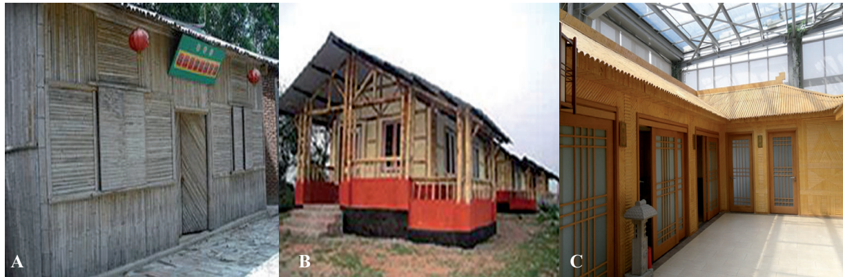
Figure 6. Bamboo houses. Traditional house (A); Traditional bahareque (B); Modern prefabricated house (C)
