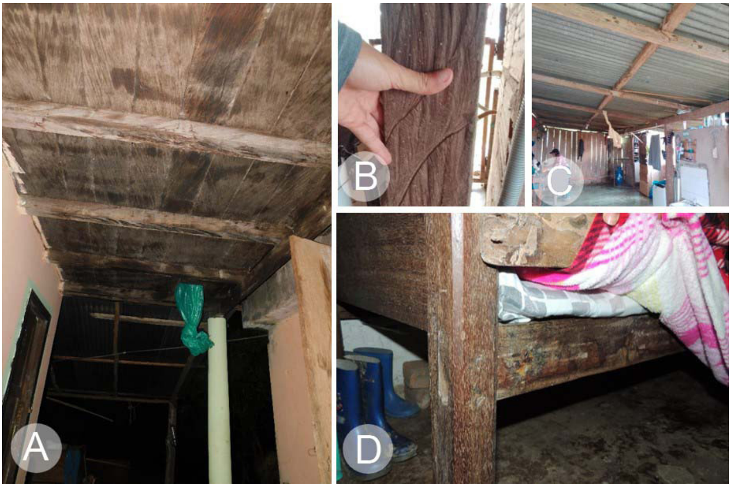
Figure 4: “Elba” house made with Caryodaphnopsis Airy Shaw wood. A. rural house supported by columns and joists of C. carmensis Humberto Mend., J. Quiroga & Díaz-Rueda; B., C., D. roof support and bed of 50 years old made with C. yariguiensis Humberto Mend., Díaz-Rueda & Aymard wood. Photographs by Daniel Díaz-Rueda.
