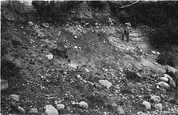
FIGURE 7.—Roadcut on St. Siméon-Chicoutimi highway  $1\frac{1}{2}$  miles from St. Siméon. Bedded sediments are overlain by gravel with boulders followed upward by till with boulders above head of man. Photograph by M. L. Miller, Quebec Dept. of Mines, No. 11592.
