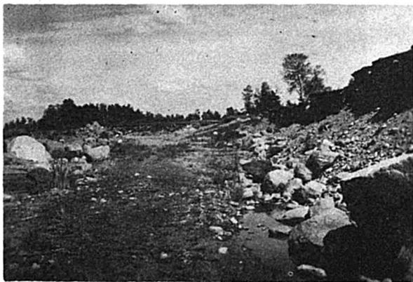
FIGURE 3.—Northeastern edge of St. Narcisse moraine showing the rapid decrease in size of the sediments. The width of the cut is the width of the gravel suitable for road construction. Silts to left of picture overlie Leda clay.
