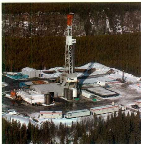
Drilling the b-60-E well at Monkman.
