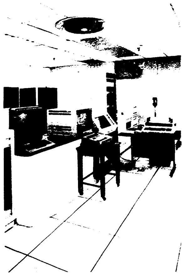
Fig. 2.4-2. Supervisory control and data acquisition development system.
