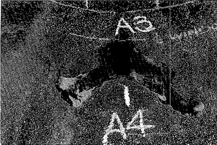
Photograph 3: Typical H.P. Pipeline corrosion cell.
