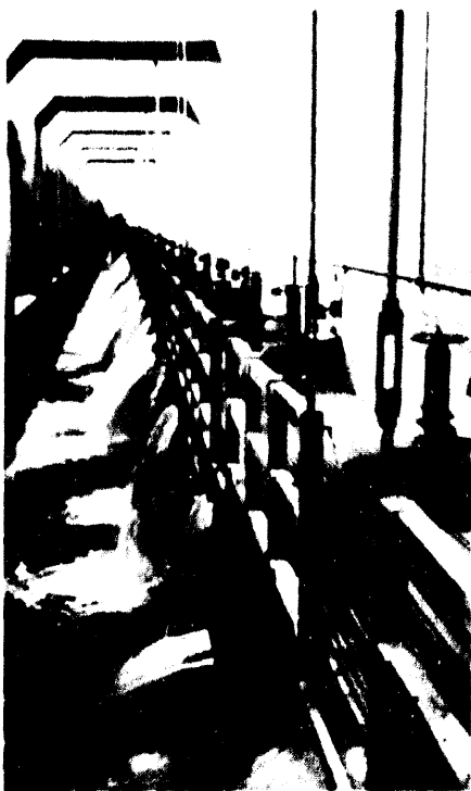
This photo depicts the 1,400-foot-long juvenile fish bypass system collection channel installed by the U.S. Army Corps of Engineers at McNary Dam. The collection channel, which is inside the ice-trash slideway, picks up fish as they exit the gatewells (the orifice valves and pipes on the right). The fish are transported to a collection facility
