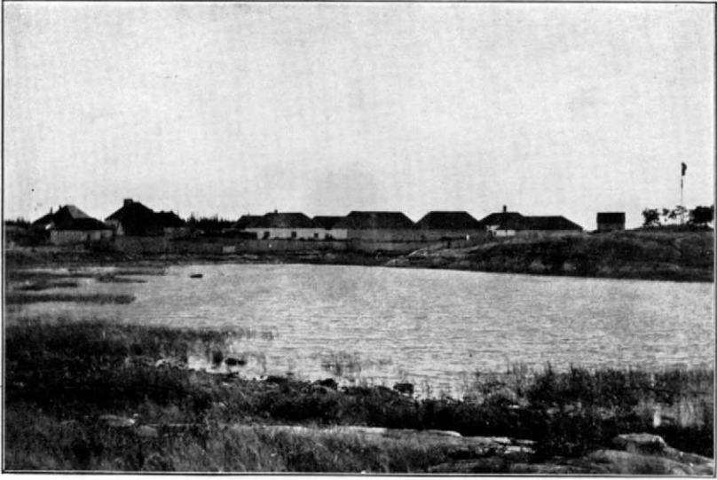
FIG. 1.—GENERAL VIEW OF NORWAY HOUSE.
