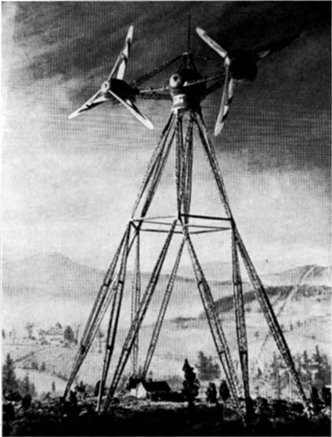
Figure 2. 7,500 kw. twin wheel turbine model
