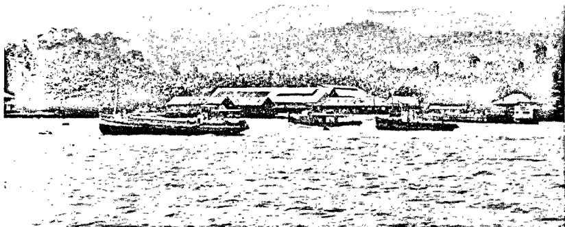
GENERAL VIEW, BOTA WHARF.
