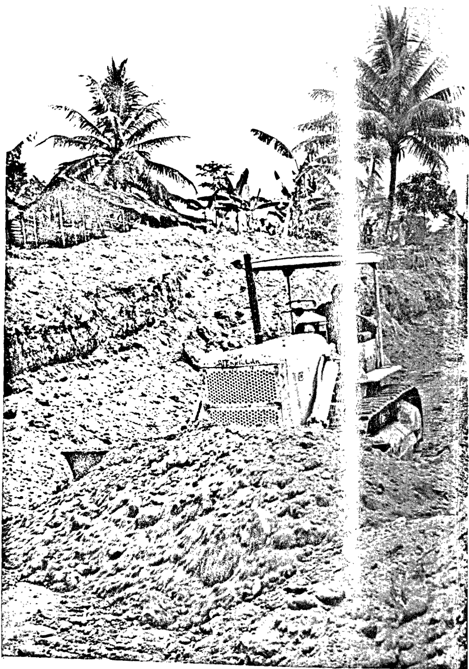
Road construction: remaking the Victoria-Kumba Road
